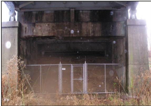
Photo 12 and 13: Bridge Design Mimicking “Cave-like” Atmosphere
