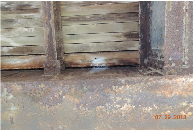
Photo 14: NLEBs Roosting Under a Timber Decked Bridge
